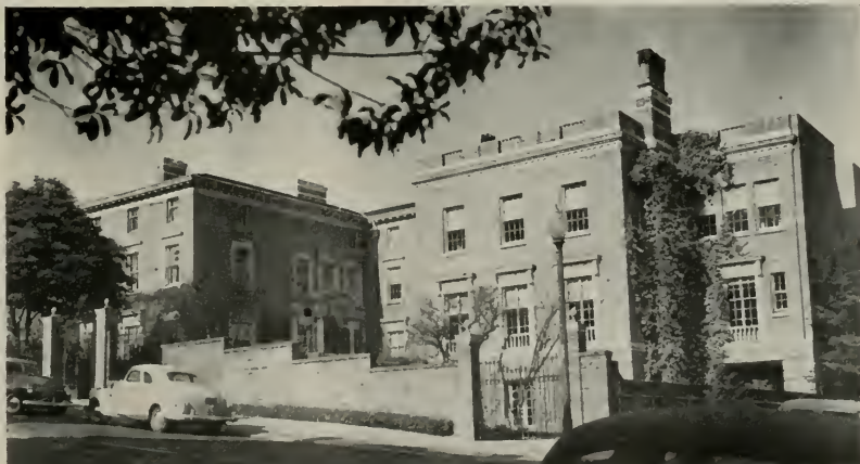
The newly acquired Swedish consulate-general in San Francisco, the former Matson mansion. A coincidence of note: Captain William Matson was the first Swedish consul in San Francisco.
